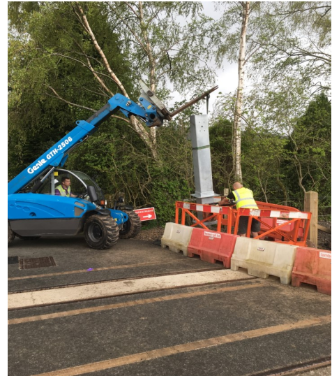
Planting a level crossing post at Slaggyford
